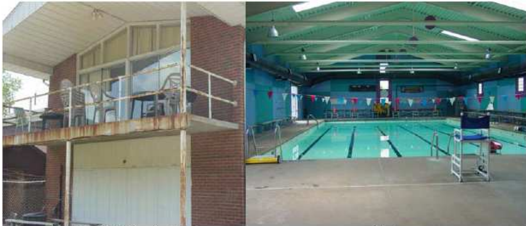
Outside of Building (backside)
